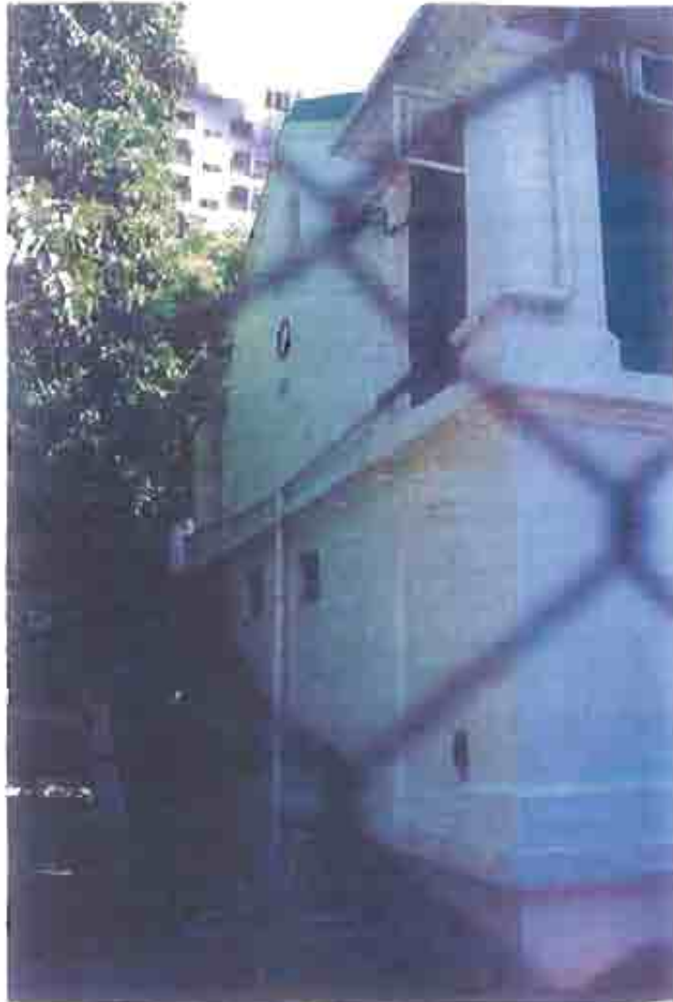
Photograph EE: Detail of east wall
