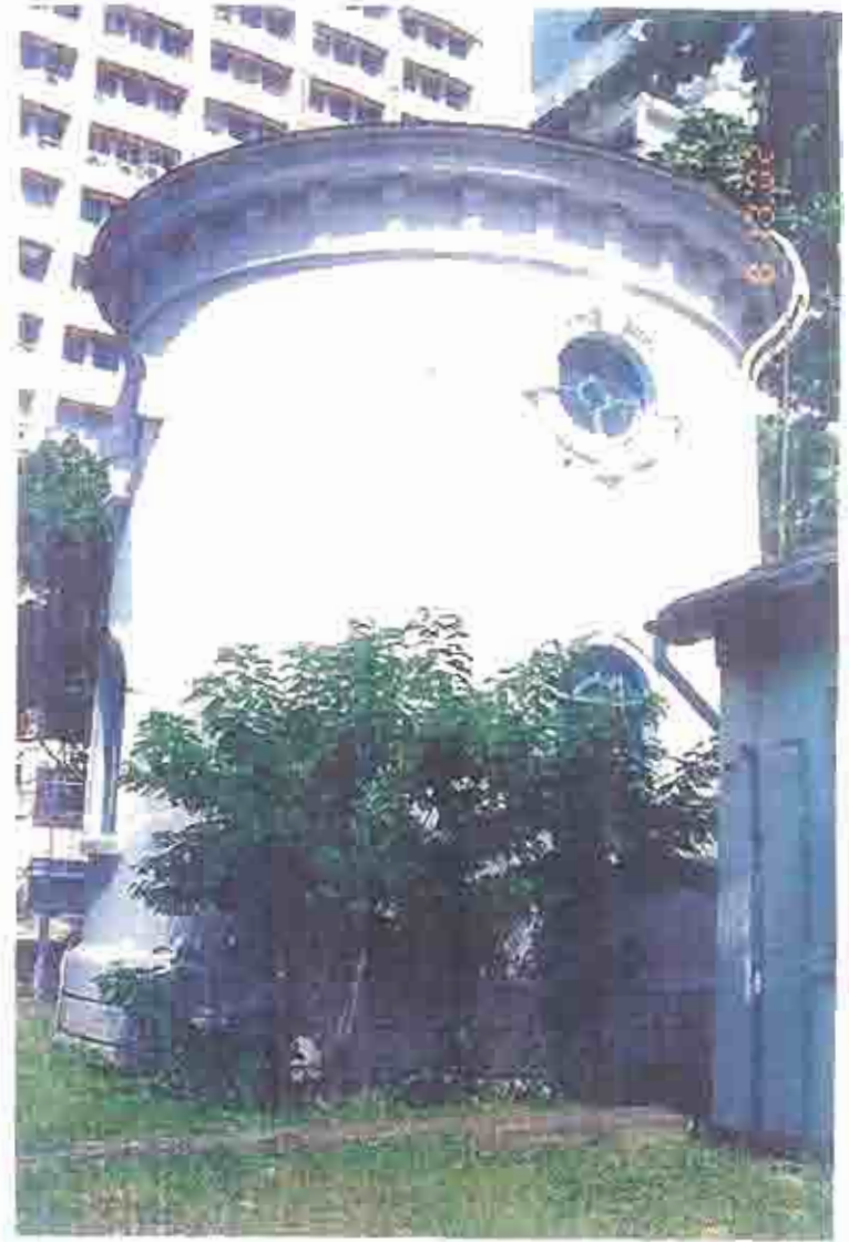
Photograph C: East facing side elevation
