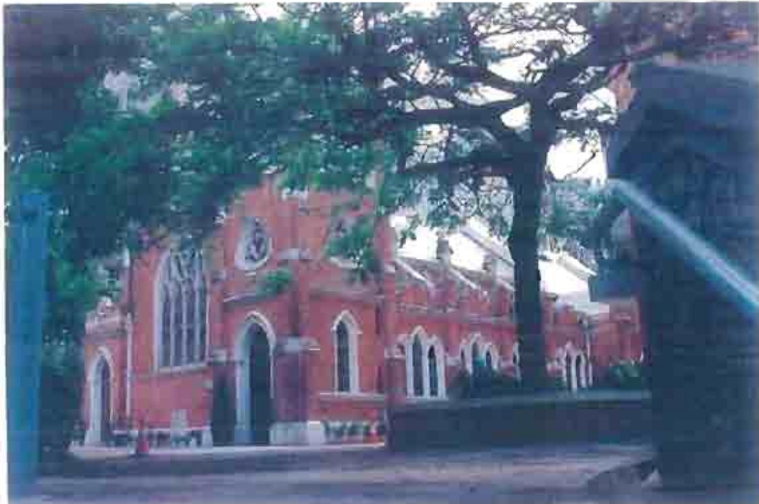
Photograph BBB: View of the church from the southwest
