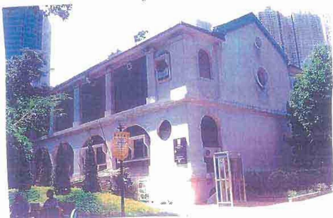
Photograph HH: View of south facing wall of S61
