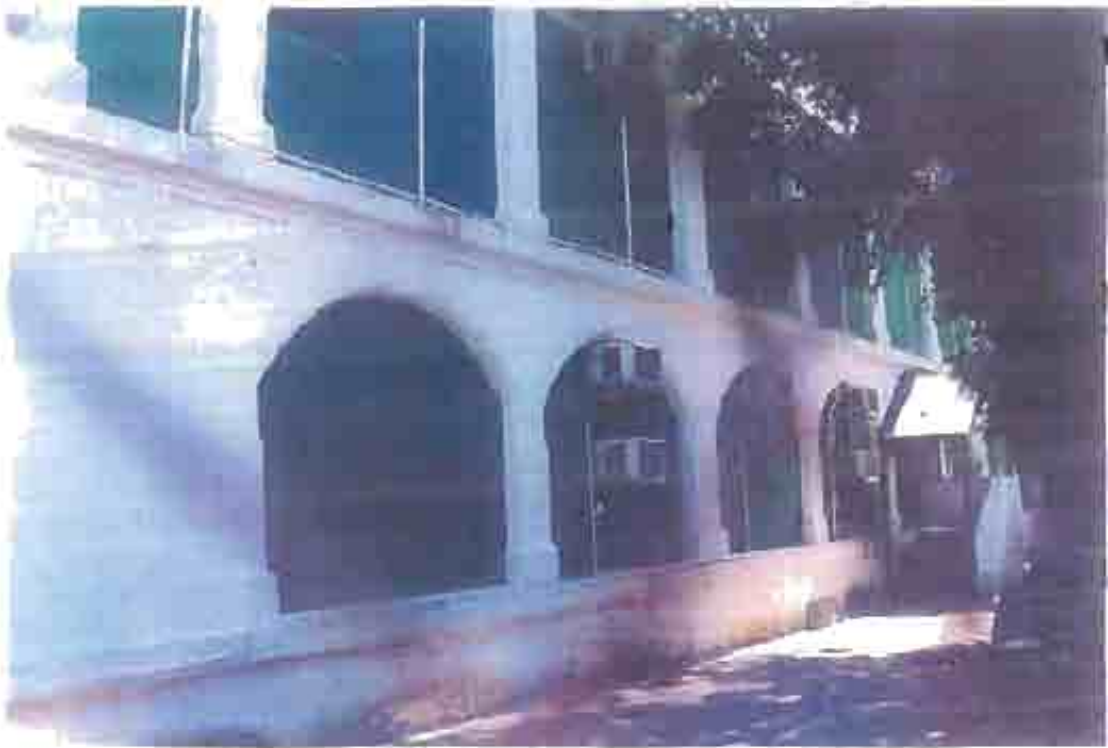
Photograph DD: View of rear wall
