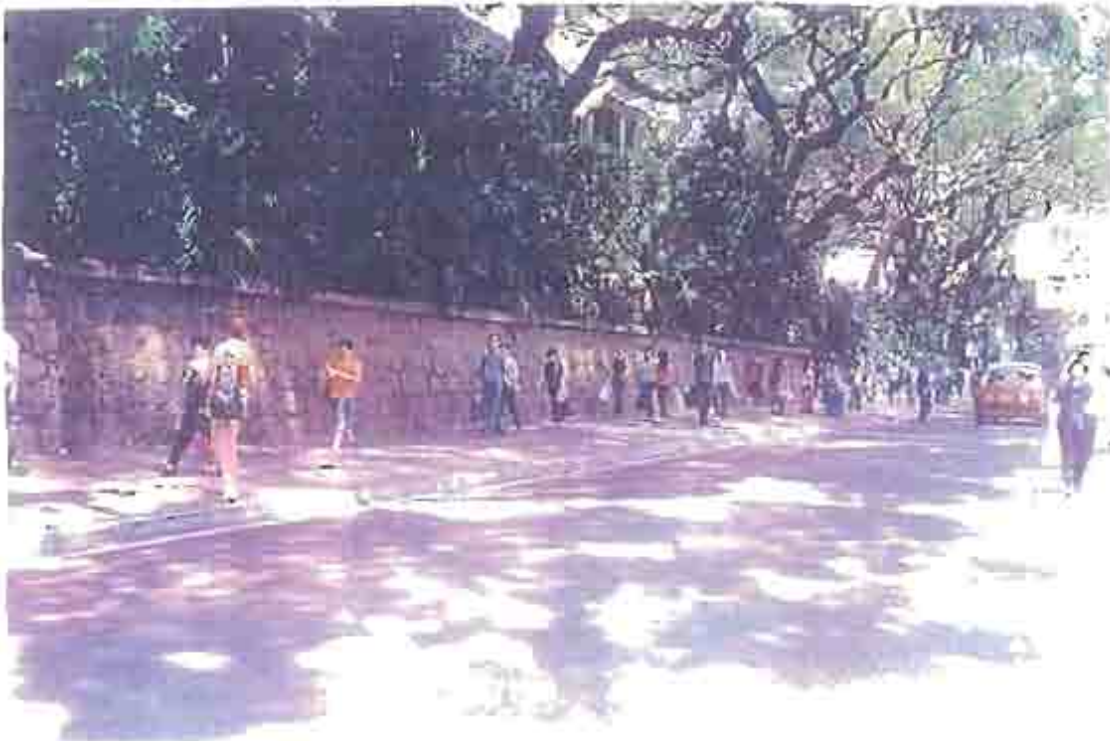
Photograph BB: View of retaining wall looking east
