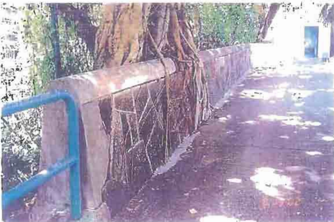
Photograph R: General view of retaining wall C
