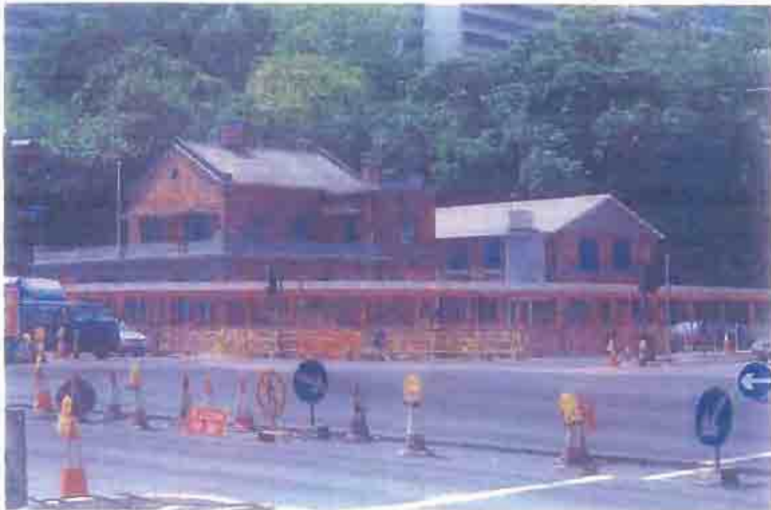
Photograph S- General view of the building
