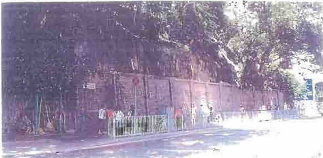
Photograph Q: General view of retaining wall B
