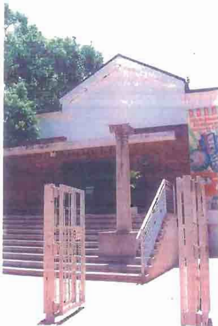
Photograph NN: View of east side of building
