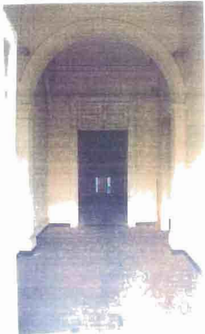
Photograph J: Detail of interior arch and doorway
