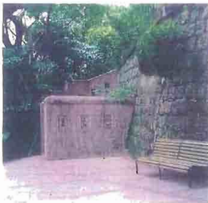
Photograph II: View of enclosure around base of steps at the west end of the wall
