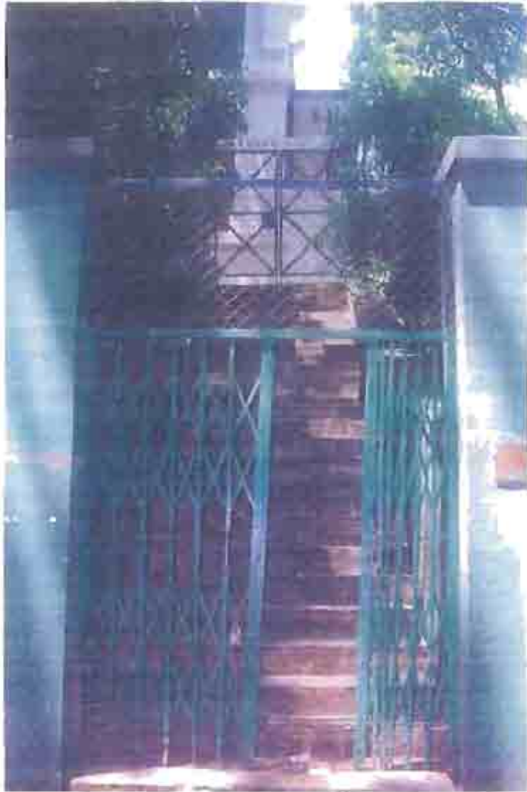
Photograph AA: Stairs leading up to Barracks building S58
