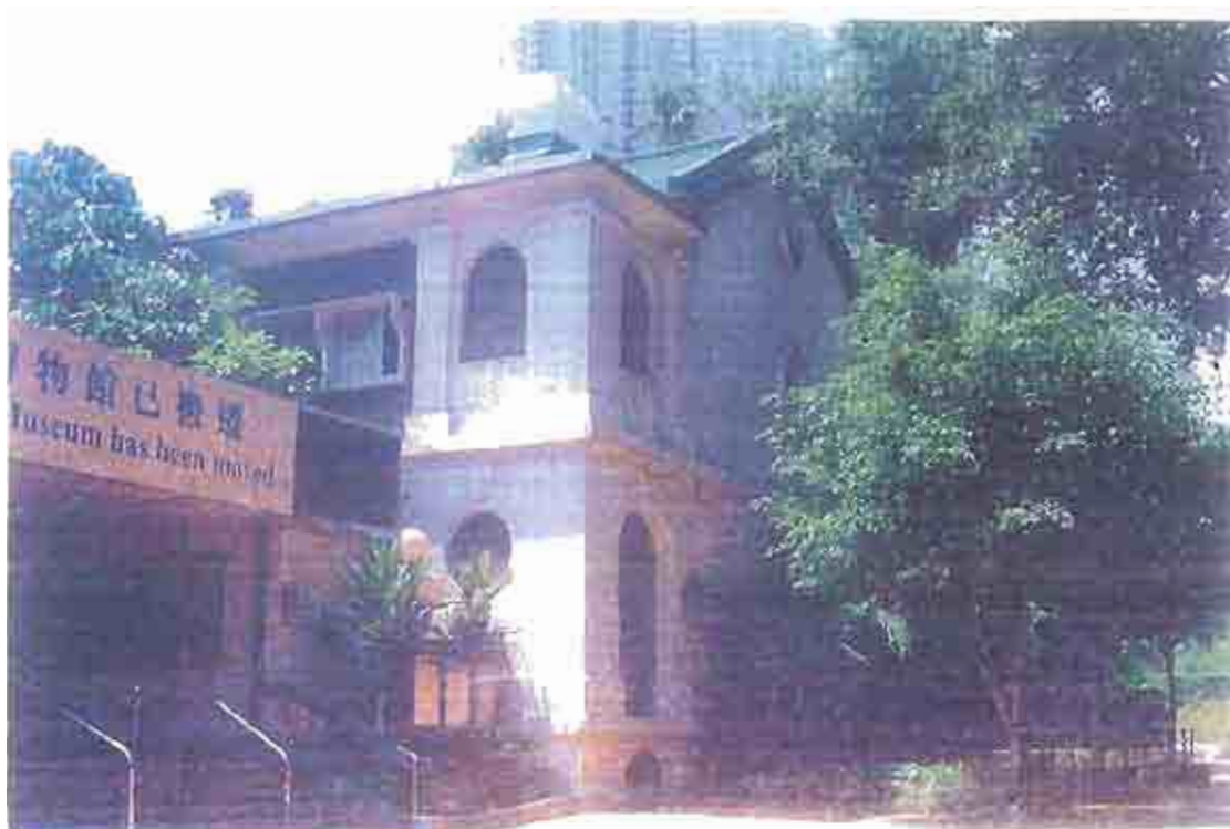
Photograph GG: View of south facing wall of S62
