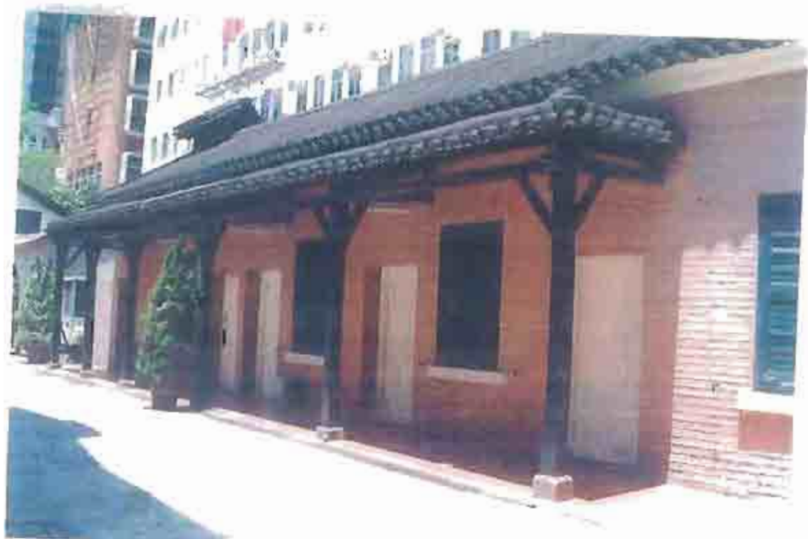
Photograph ZZ: Front view of the rear block
