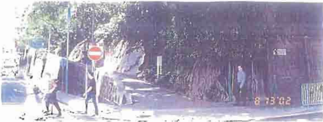
Photograph P: General view of retaining wall A
