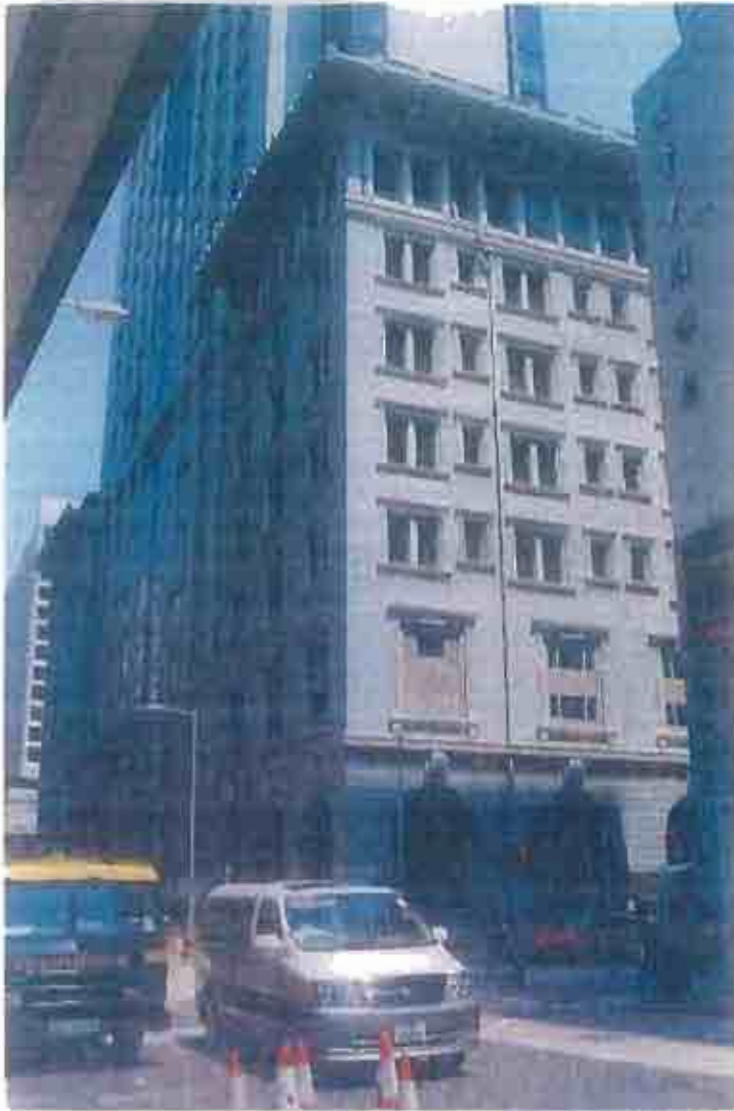
Photograph QQ: View of the rear of the building from the west
