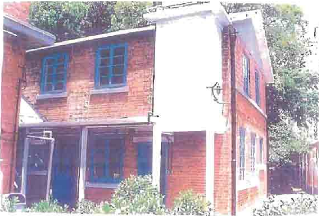
Photograph T: View of south side of building
