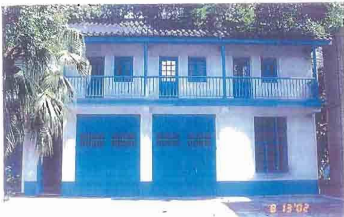
Photograph A: Front Elevation
