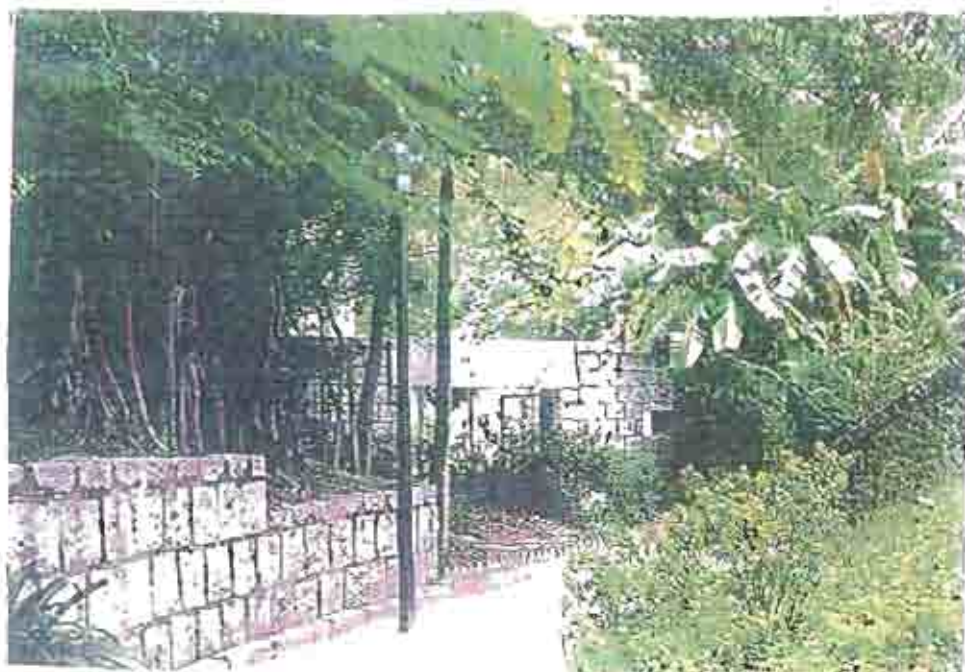
Photograph KK - View of cut stone walls
