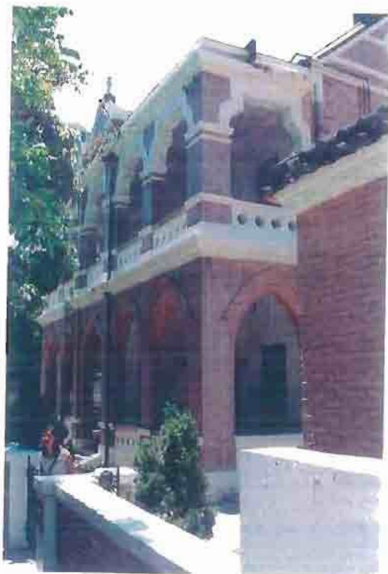
Photograph AAA: View of the south wall
